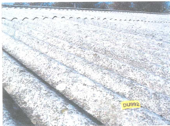
Corrugated asbestos cement roof
